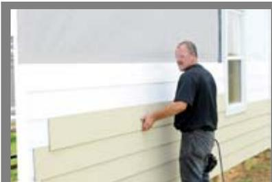
Installing siding on a building frame where exterior insulation has been applied takes special care to make sure the cladding gets properly attached to the frame. *(Photo courtesy of Progressive Foam)*
